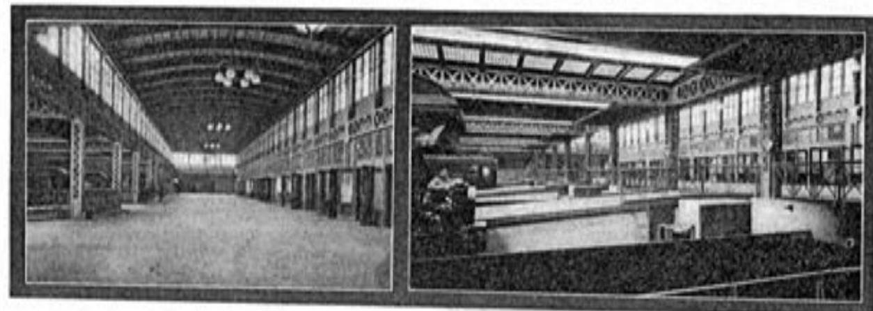
The South Train Concourse—Passenger Platforms Are Connected to the Train Concourse Floor by Means of Ramps Enclosure for One of the Baggage Platform Ramps in Foreground
