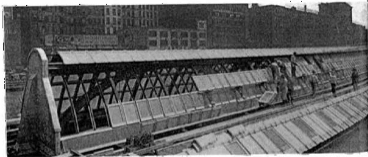
The Concrete Tile and Glass Block Were Made to Fit Accurately to the Steel Frame of the Train Sheds.
